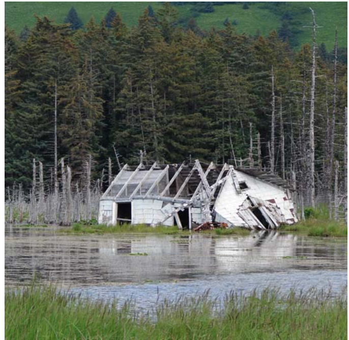
A home destroyed on Afognak Island from the 1964 tsunami
